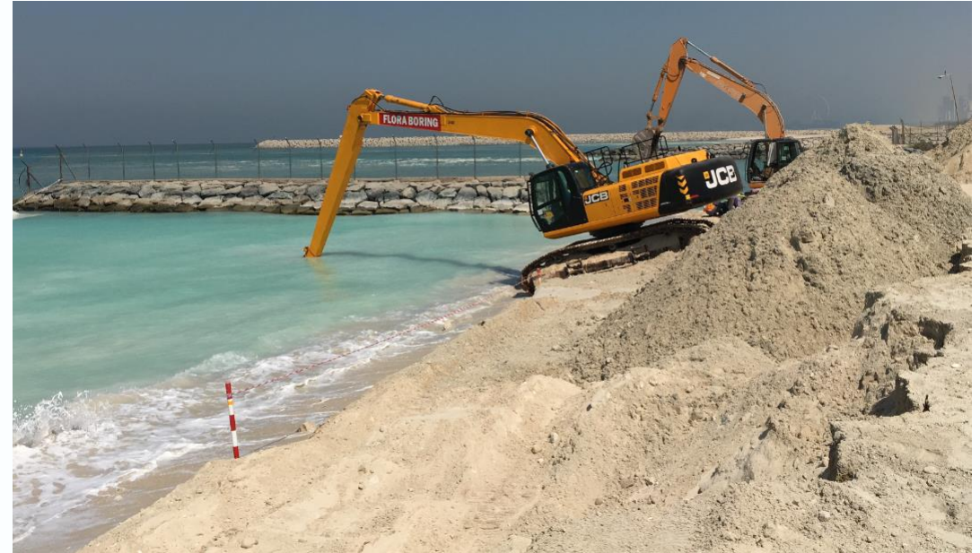
Toe trench excavation
